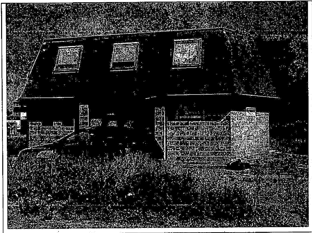
Plate 1. The Existing Building on the Application Site.
