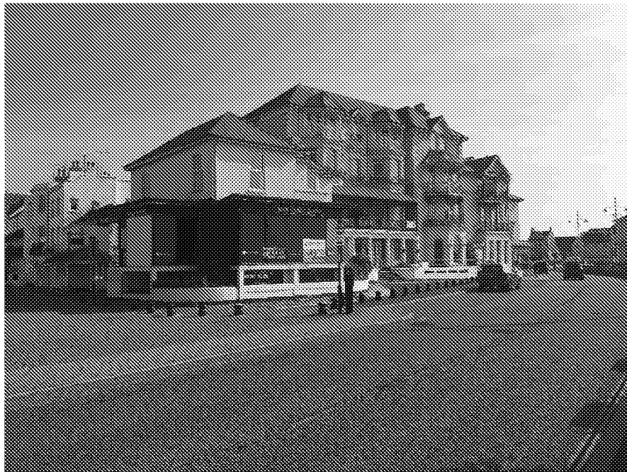
Application site viewed from the Esplanade seafront
