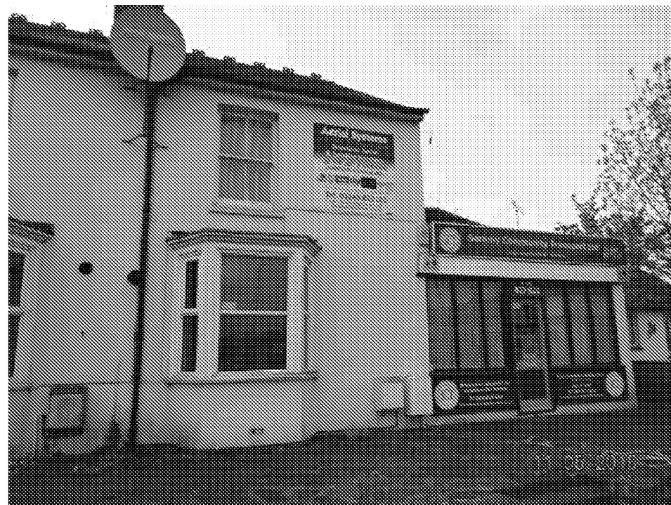
North, front elevation of 285 Chichester Road
