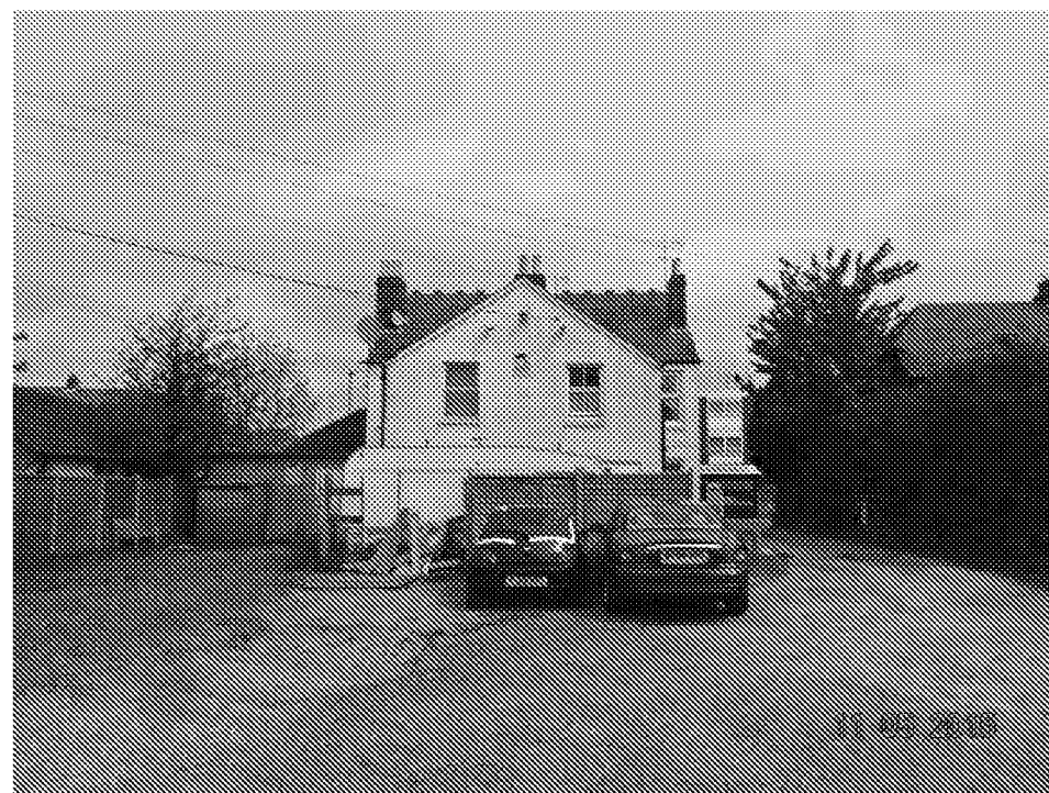
View looking north to rear of 283-286 Chichester Road
