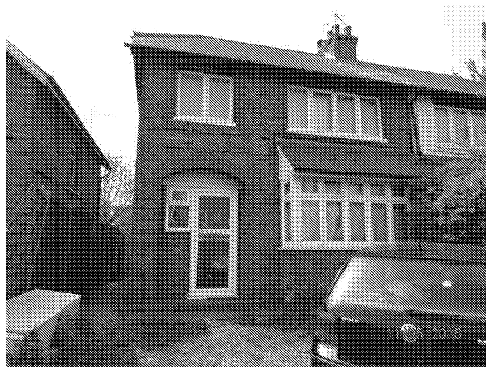
North, front elevation of 279 Chichester Road
