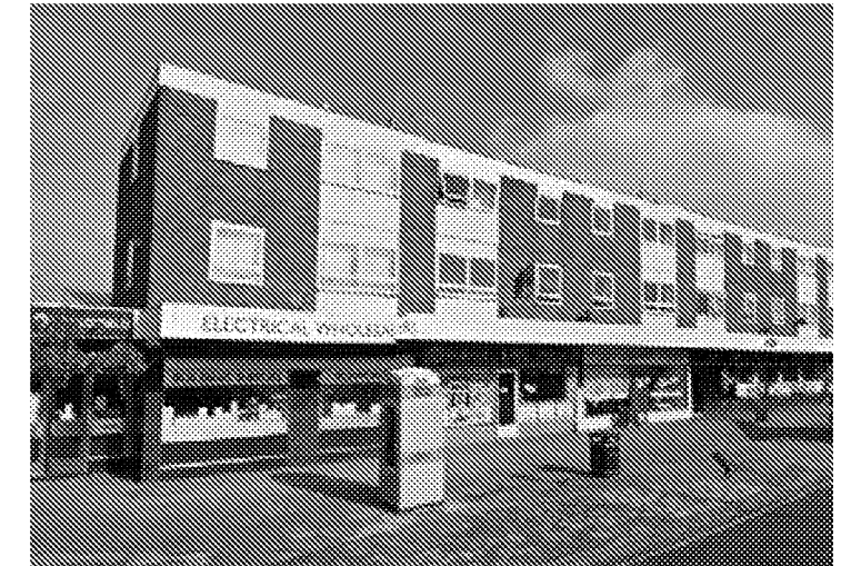
Three storey parade opposite site
