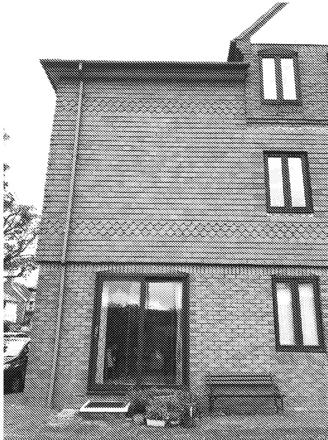
Photo 4 – External North East Elevation - Block B - Elevation 3
