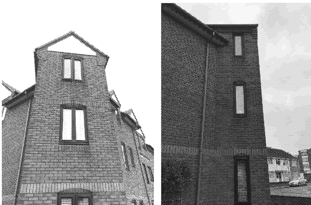
Photo 3a + 3b External South Elevation – Block A – Elevations 1,2 and 3
