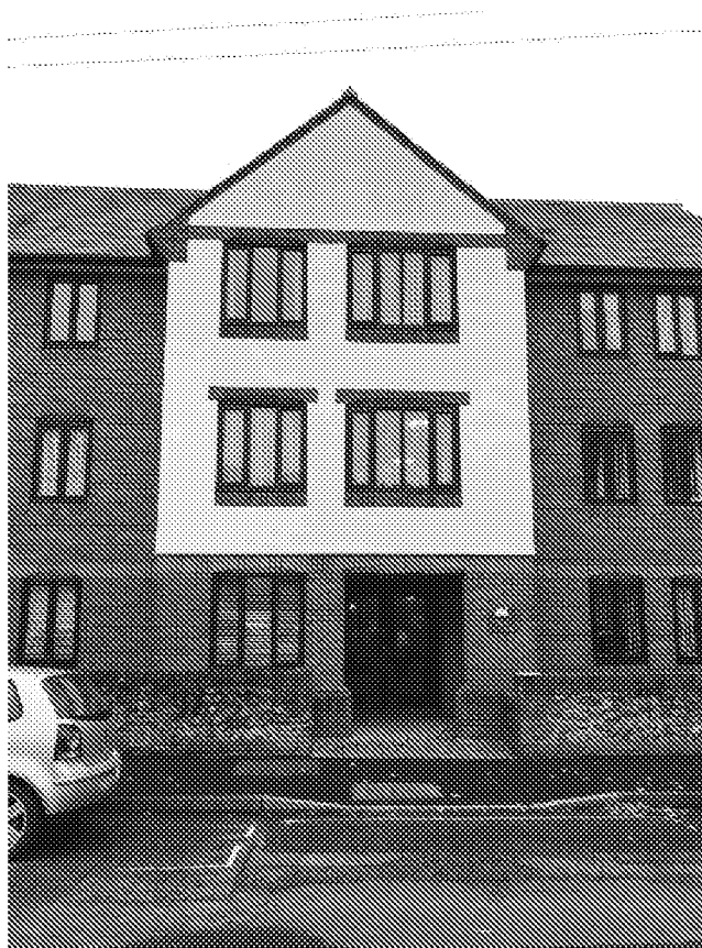
Photo 2: External South West Elevation — Block B – Elevation 1
