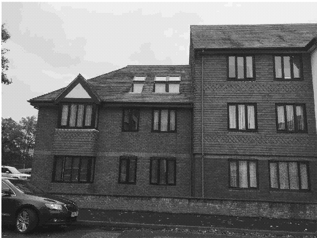
Photo 1a + 1b: External South West Elevation – Block A - Elevation 1
