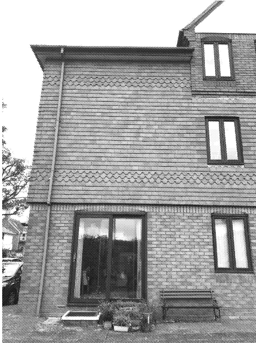
Photo 4 – External North East Elevation - Block B - Elevation 3
