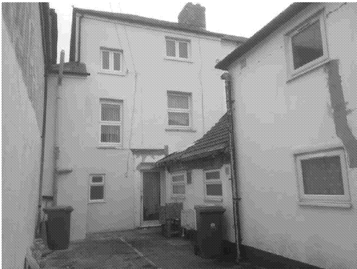
Rear courtyard of 9b Waterloo Square
