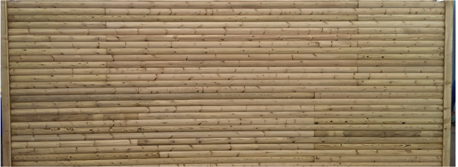
Figure 1. Bare timber cladding to shipping container.
