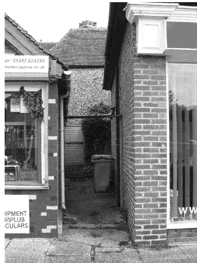
(06) Photo looking north along the shared side footpath access, towards the rear courtyard area, highlighting its existing proportions and the nature of the existing surface water gully arrangement.
