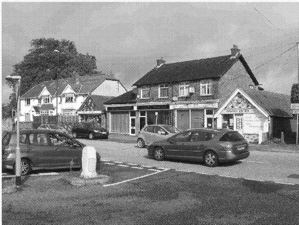
(03) Photo looking North at the junction of Hawthorn Road and Chichester Road, highlighting the material character, form, composition and scale of No's, 94, 96, 98, 100 and 102, relative to each other.
