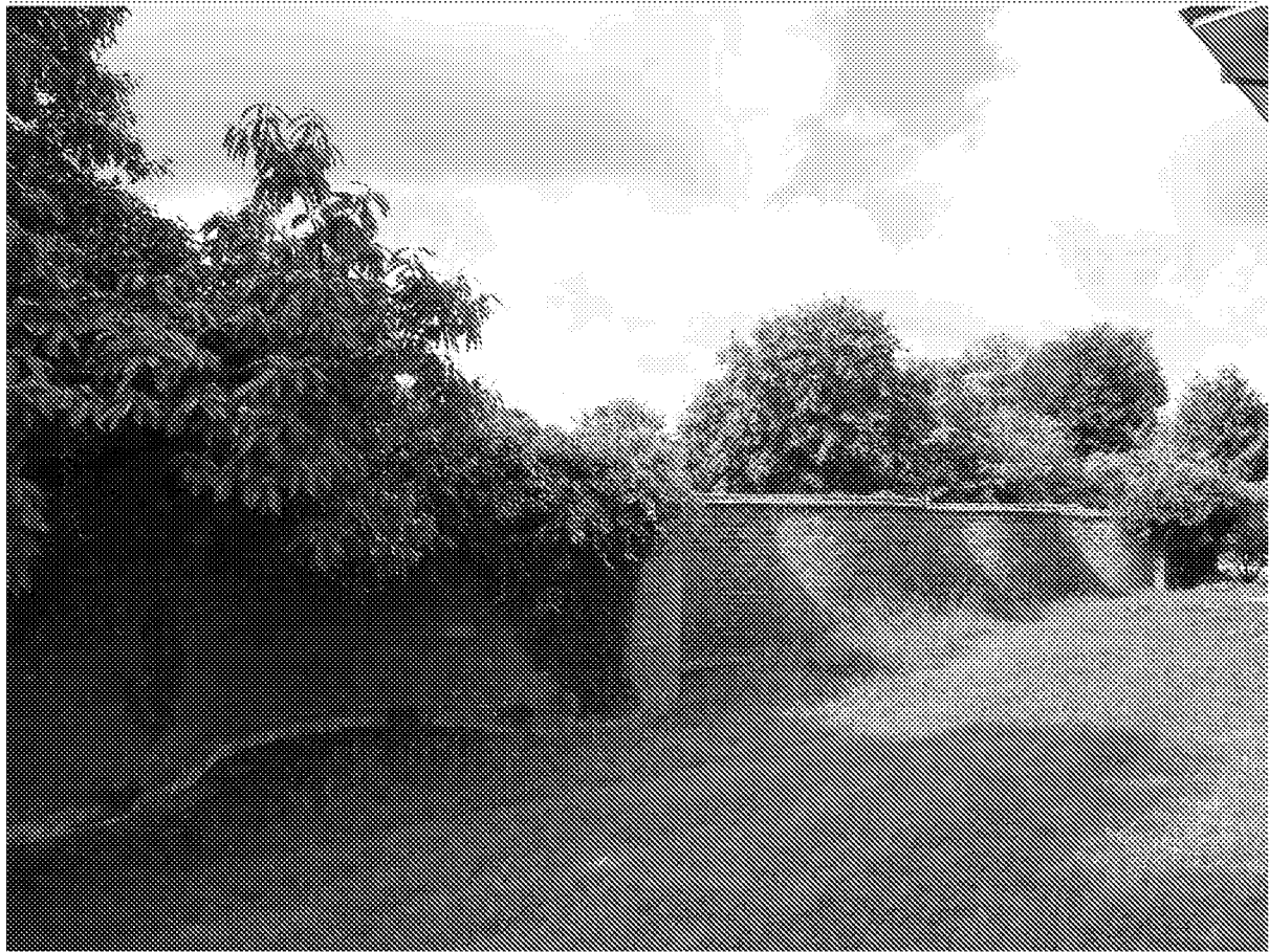
Figure 17: Serpentine wall – north elevation
