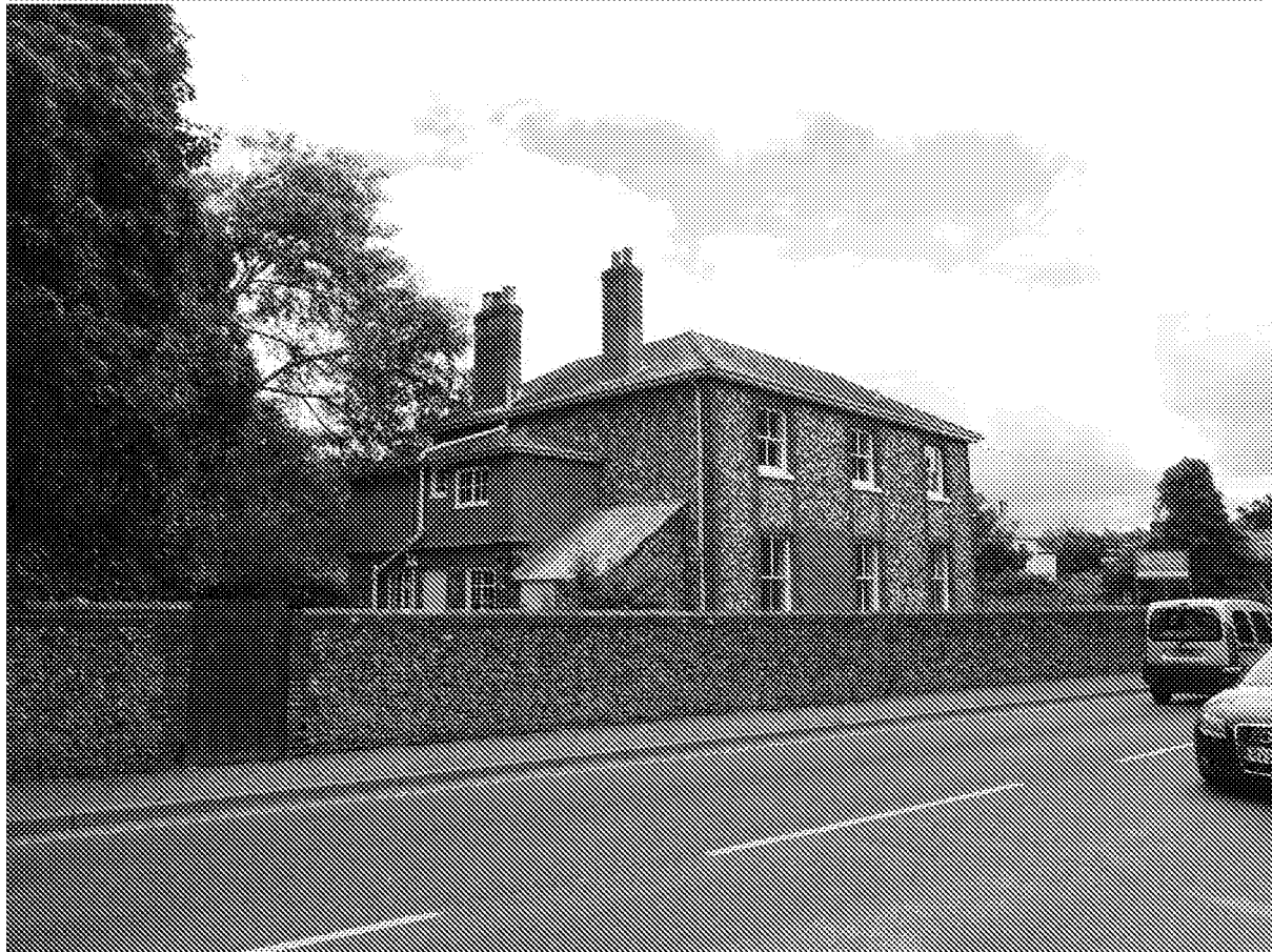
Figure 5: No.65 Upper Bognor Road – south elevation
