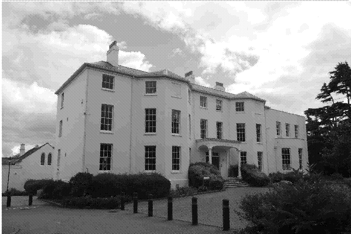
Figure 3: No.57 St Michael's House, Upper Bognor Road – south elevation
