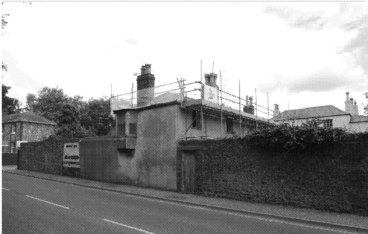
Figure 7: Nos 67 and 69 Upper Bognor Road – south and part east elevations
