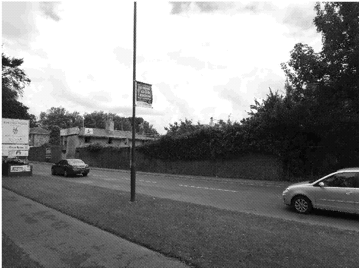
Figure 8: Boundary wall to Nos. 67 and 69 Upper Bognor Road
