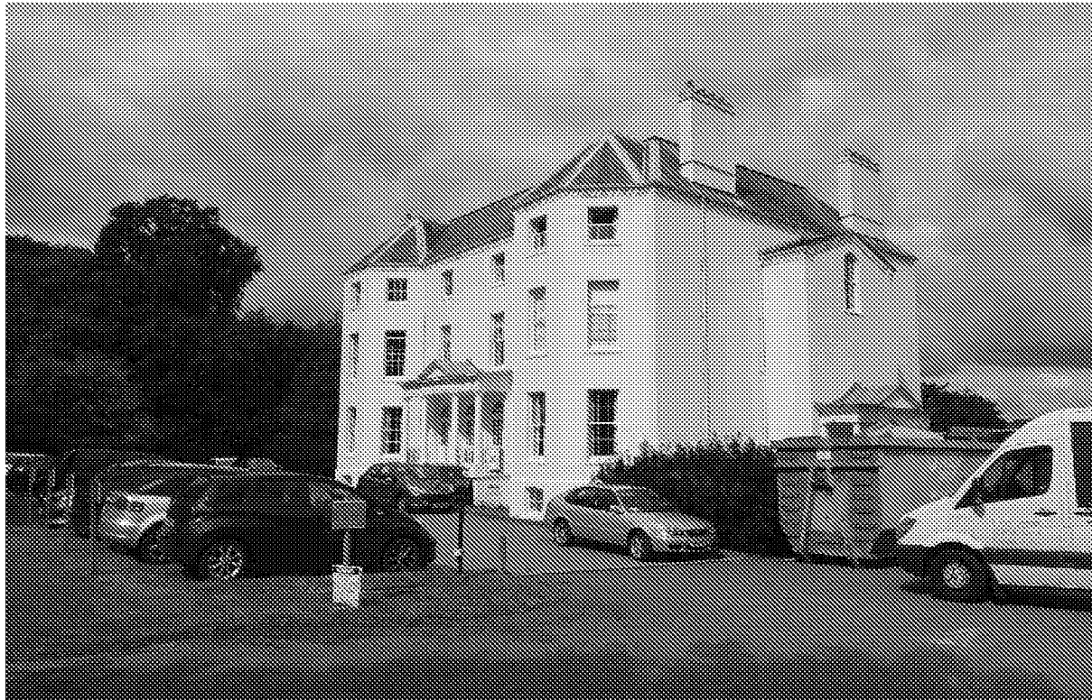
Figure 1: No.53 Mordington, Upper Bognor Road – south elevation
