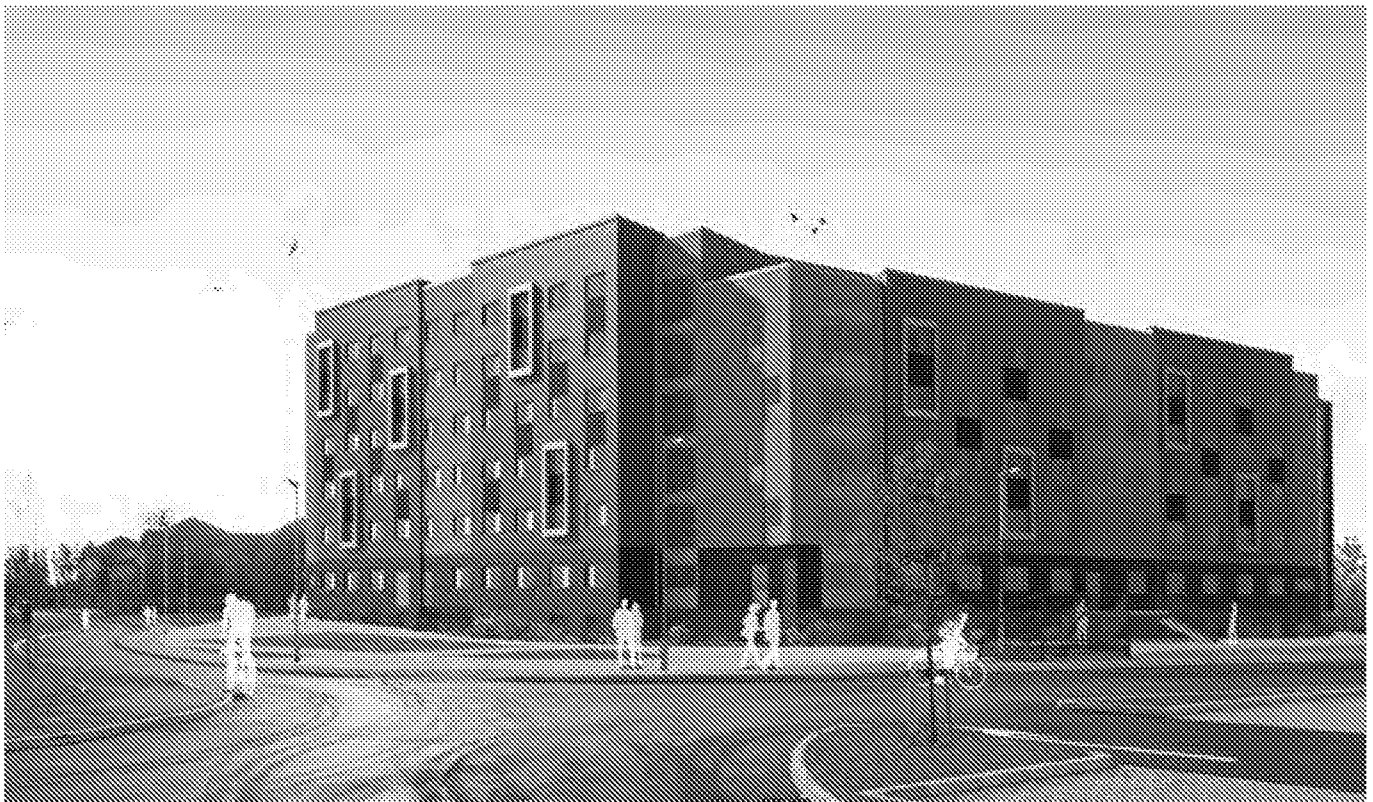
Fig 02: Proposed student accommodation building from the Tech Park access road and car park to the north-east
