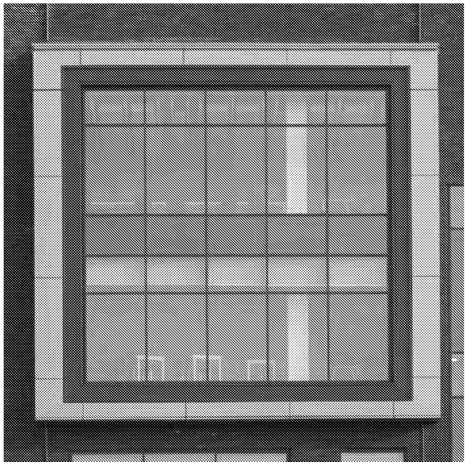
Fig 45: Protruding framed windows at Tech Park, in gold cladding
