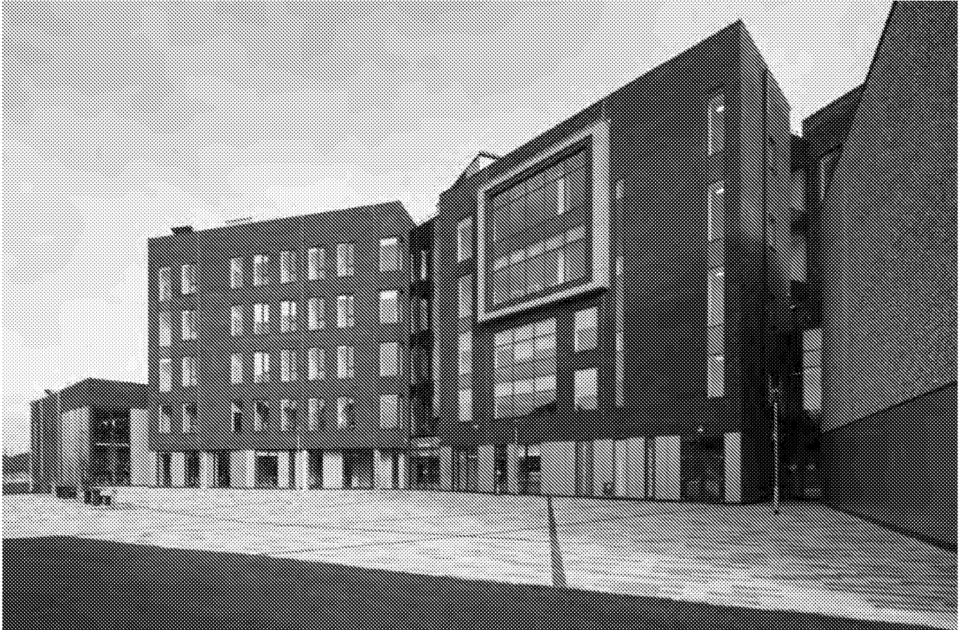
Fig 40: Recently-completed Tech Park academic building - entrance and courtyard - dark brick, gold cladding, flint
