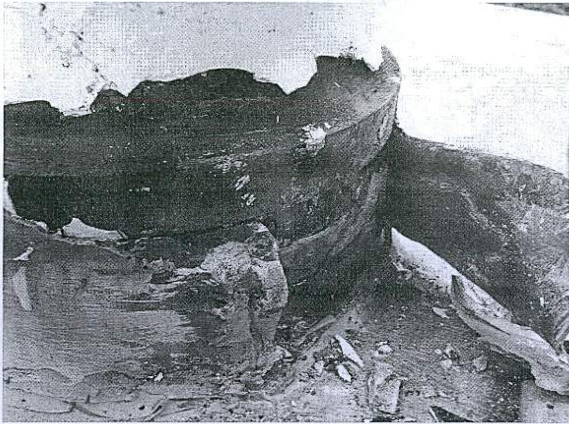
6) outer lead collar removed exposing rebate and welded upstand
