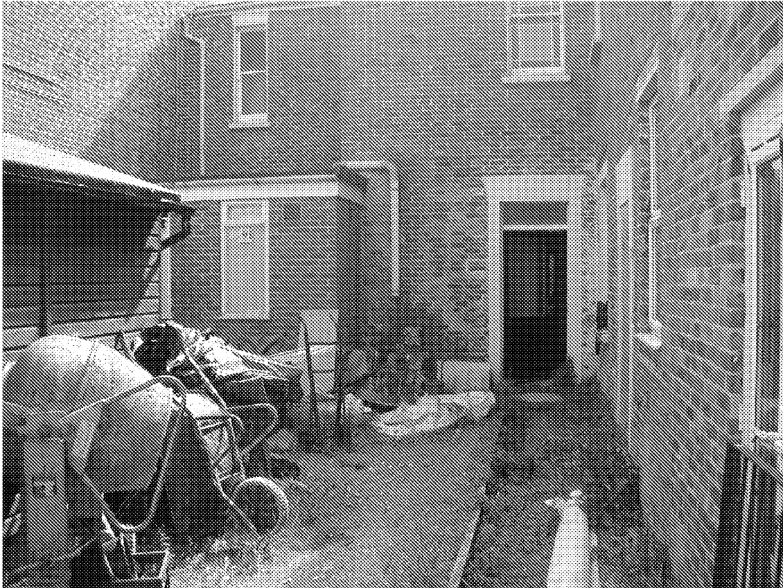
Picture – Rear of the building as it exists.
