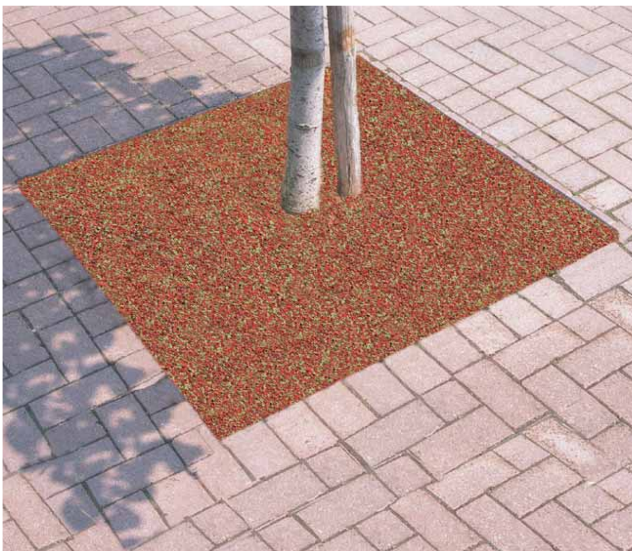
ECOFILL™ used solely within a tree well to create a tree grille within a block paved area.
