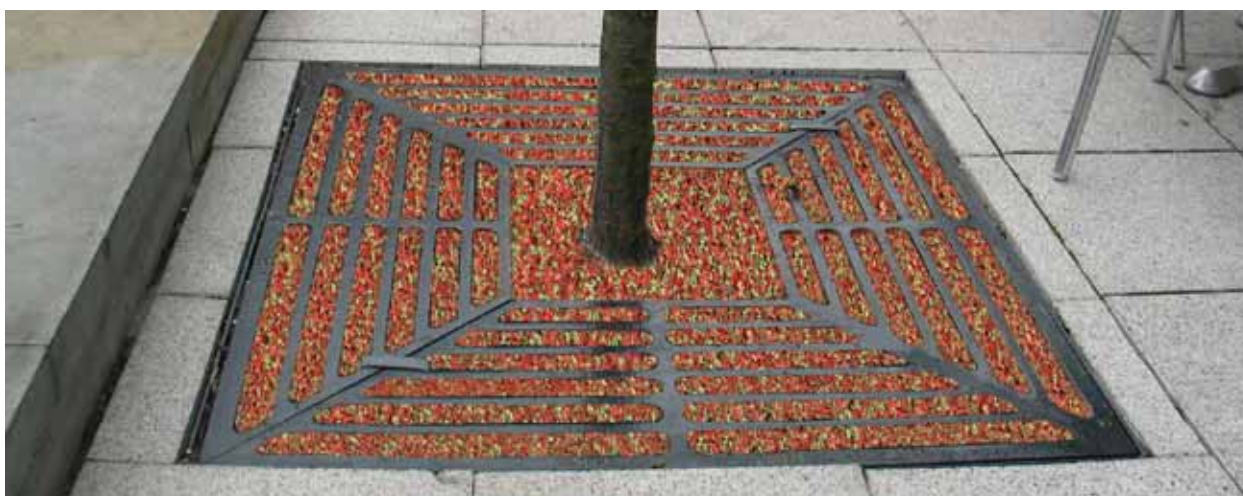
Broxap's standard BX436-1 Kings Lynn tree grille retro-fitted with ECOFILL™
