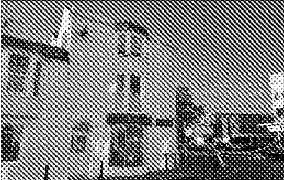
Plate 7: Nos. 61 to 65 High Street (centre & centre left) shown relative to Nos. 2-10 Queensway (ringed)
