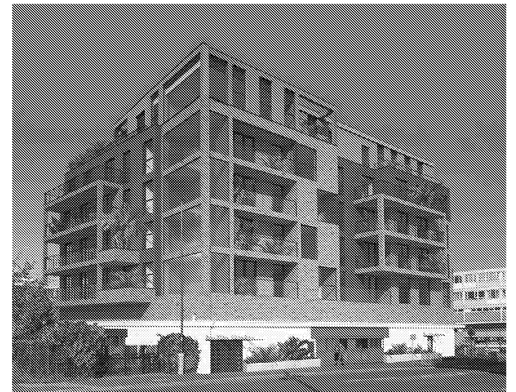
STREET VIEW PEDESTRIAN VIEW LOOKING NORTH-EAST
