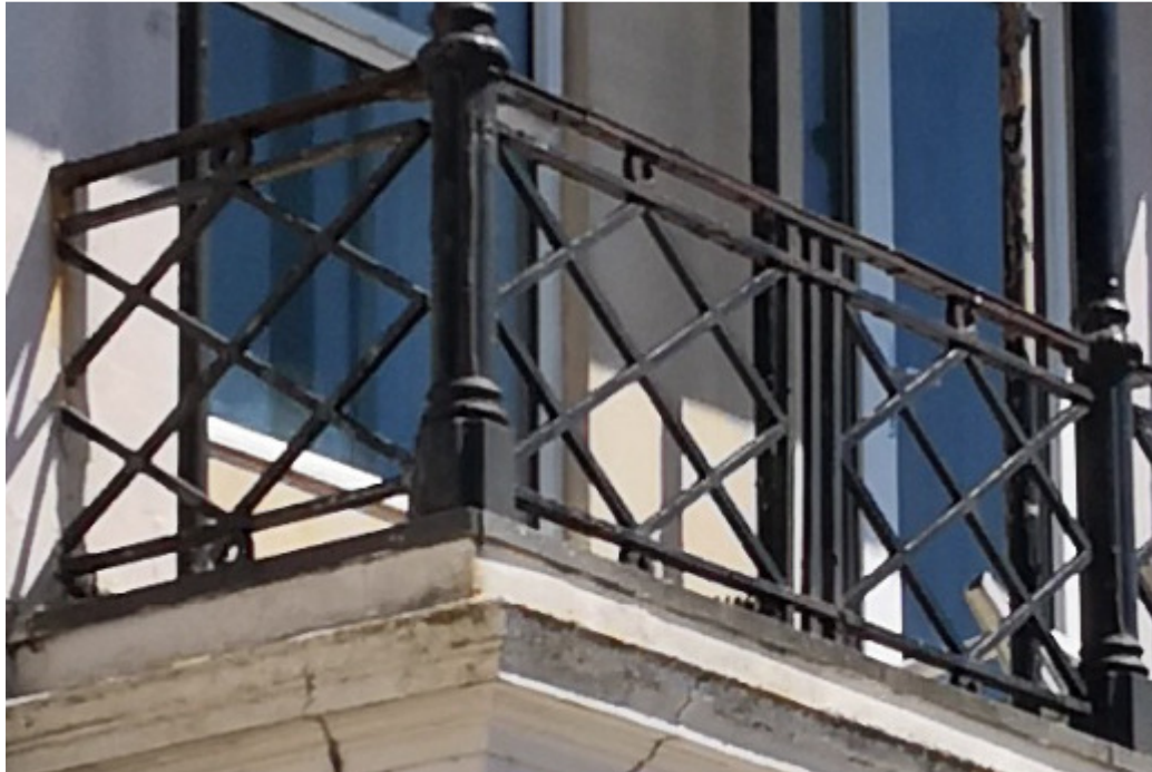
Photograph of existing metalwork, pre-refurbishment
