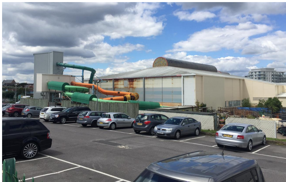
Former swimming pool building - Butlins Resort, Bognor Regis
