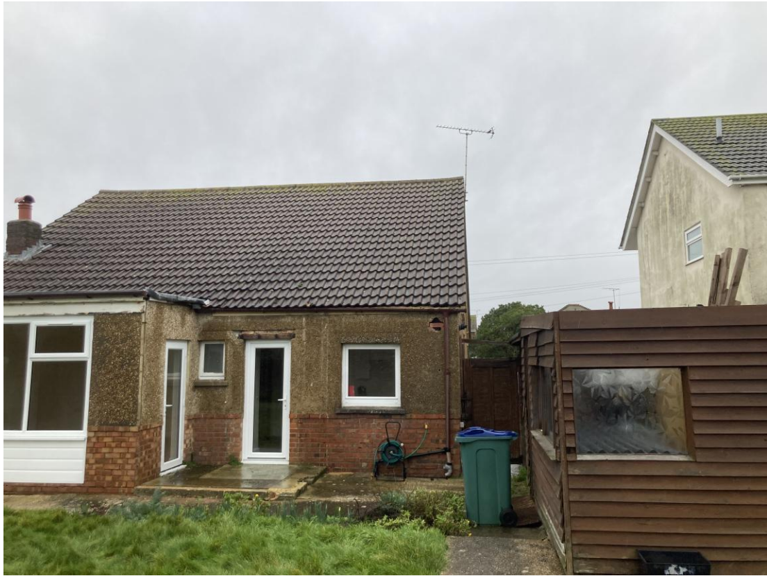
Photograph 03 – Showing the existing Rear Elevation.
