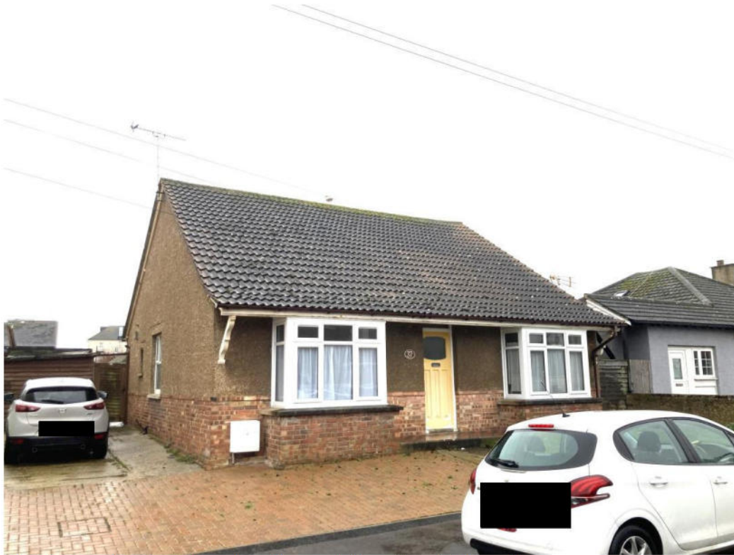
Photograph 01 – Showing the existing Front Elevation.
