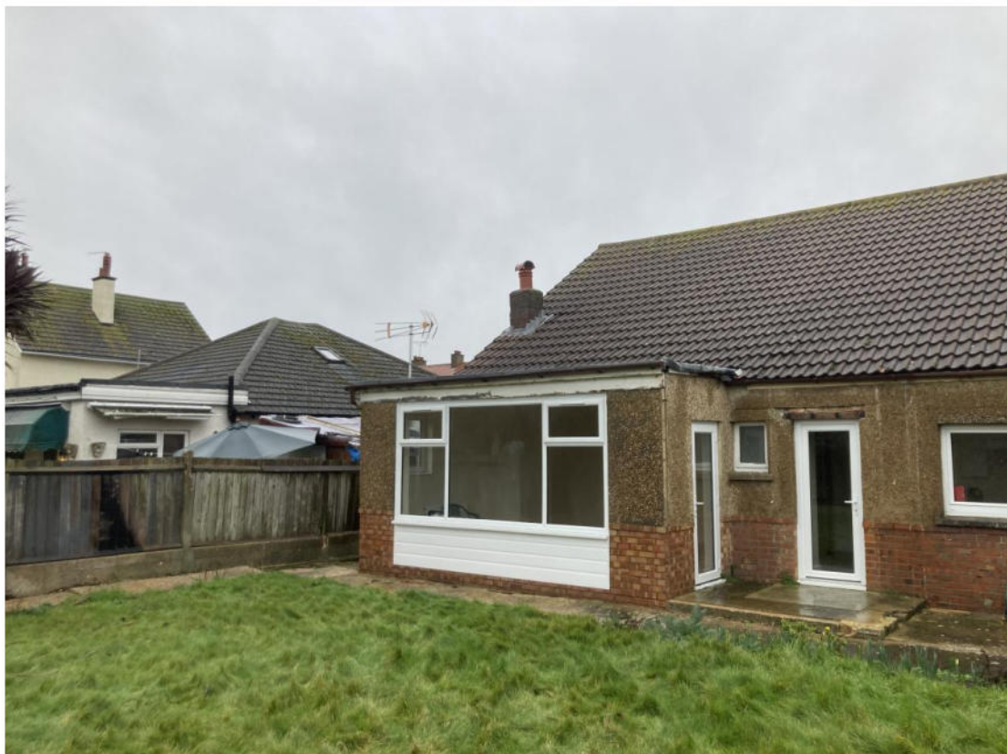
Photograph 02 – Showing the existing Rear Elevation.
