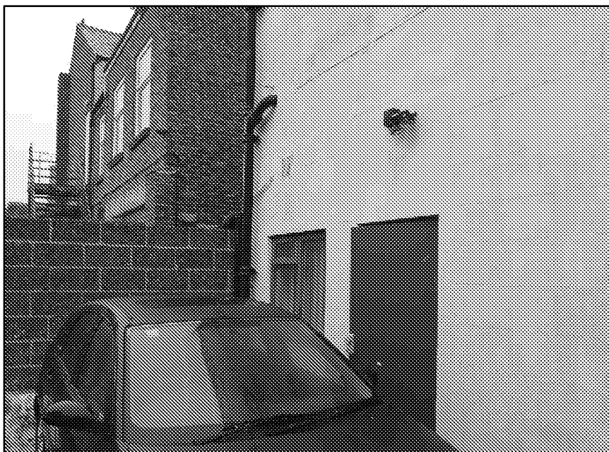
Existing door and window to rear of property
