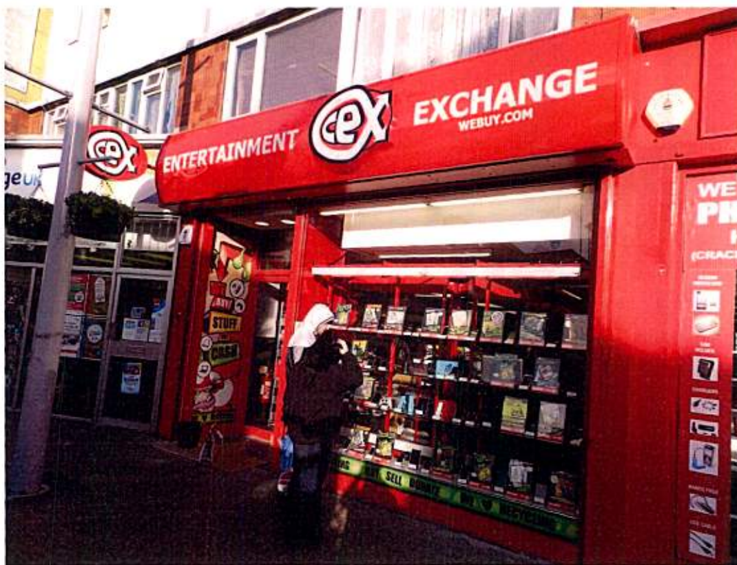
Shopfront & shutter as of 10.12.14
