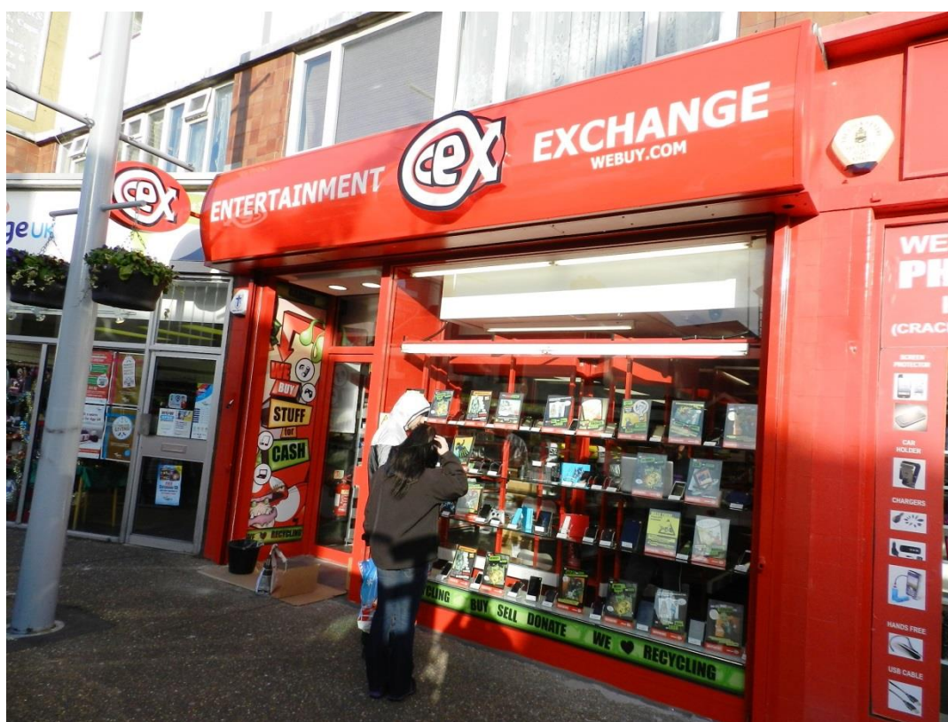
Shopfront & shutter as of 10.12.14
