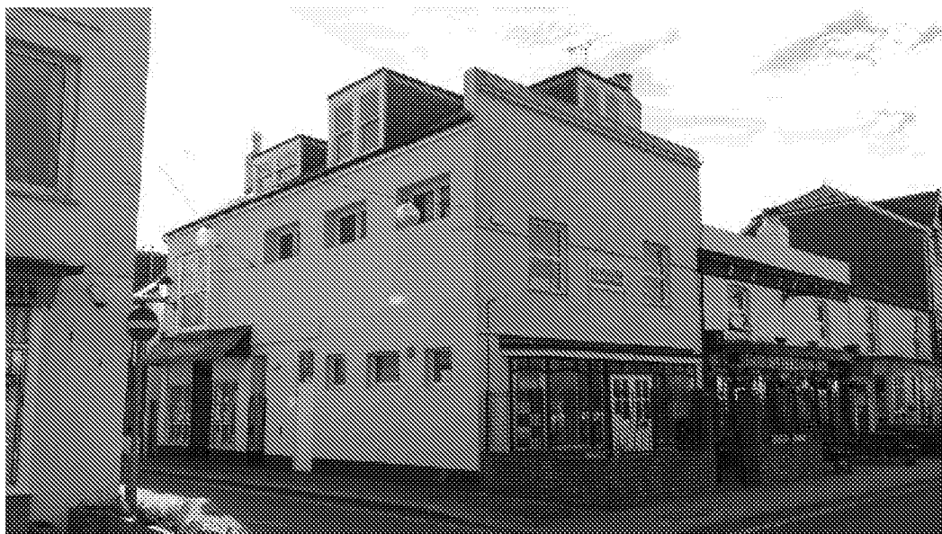
The site viewed from Waterloo Square
