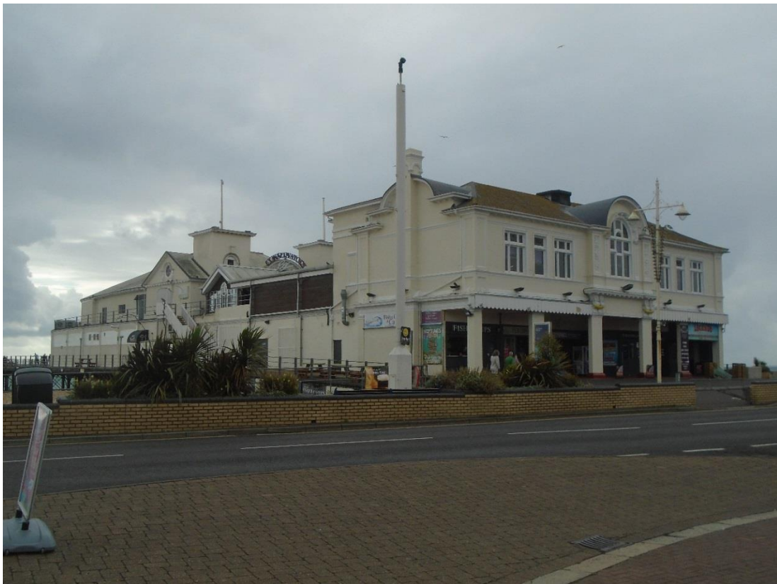
Figure 8. Bognor Pier as existing.
