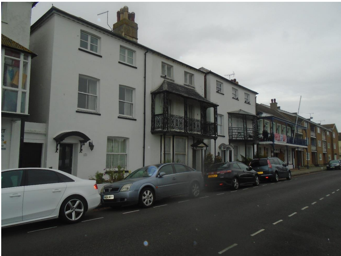
Figure 6. Nos. 7-17 Waterloo Square
