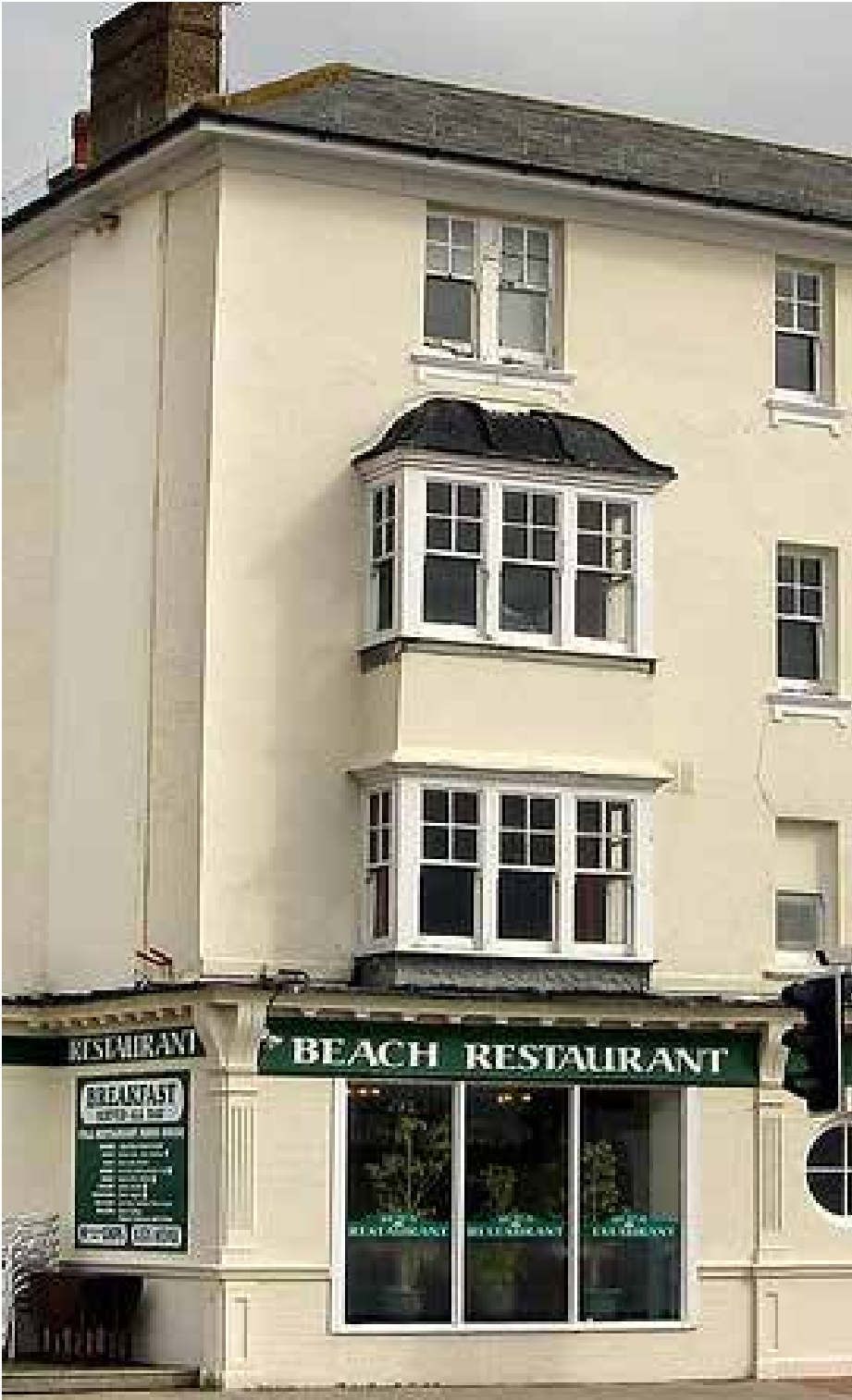
The Former Beach Hotel before demolition
