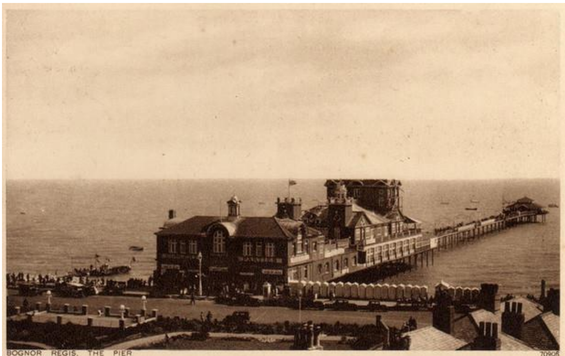
Figure 7. Late 19 th century view of pier.
