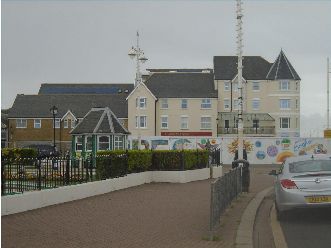
Figure 2. Current view of site looking through to Norfolk Street.
