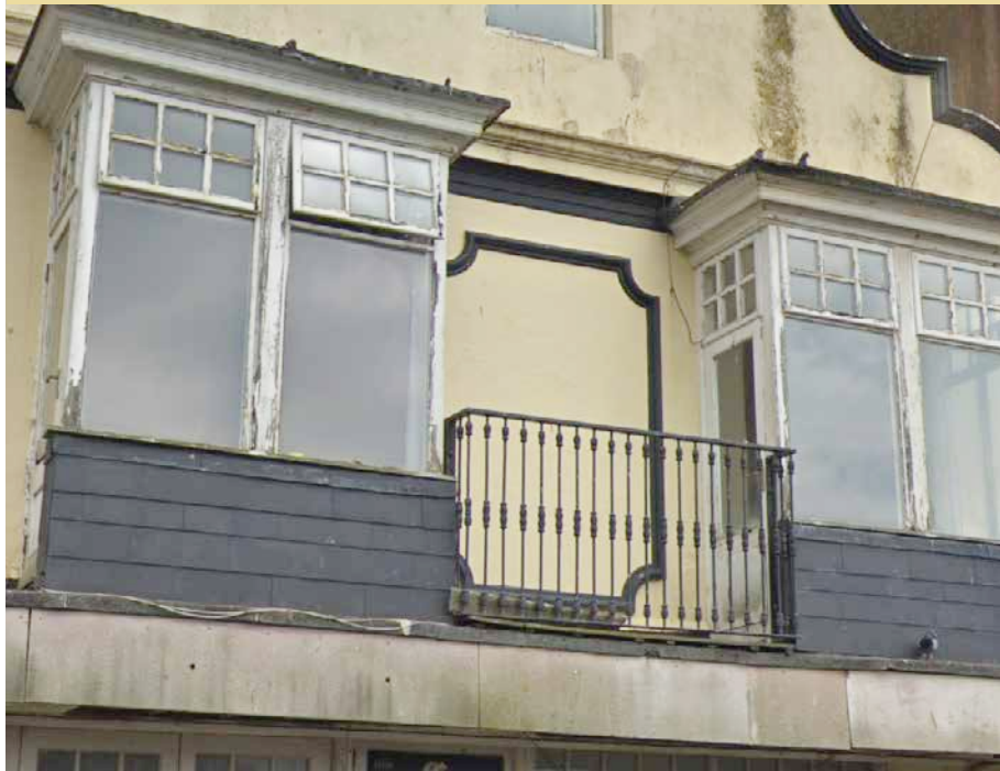
4 Waterloo Square, PO21 1SU
