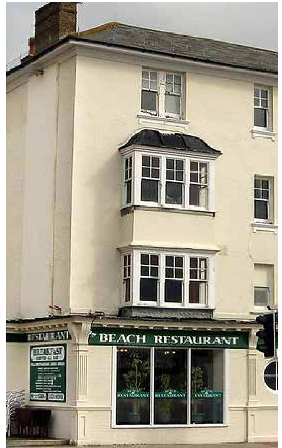
The Former Beach Hotel before demolition
