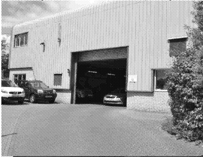
Figure 4: Front entrance and parking
