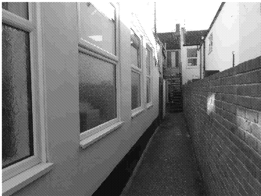
5 – Gated side access
