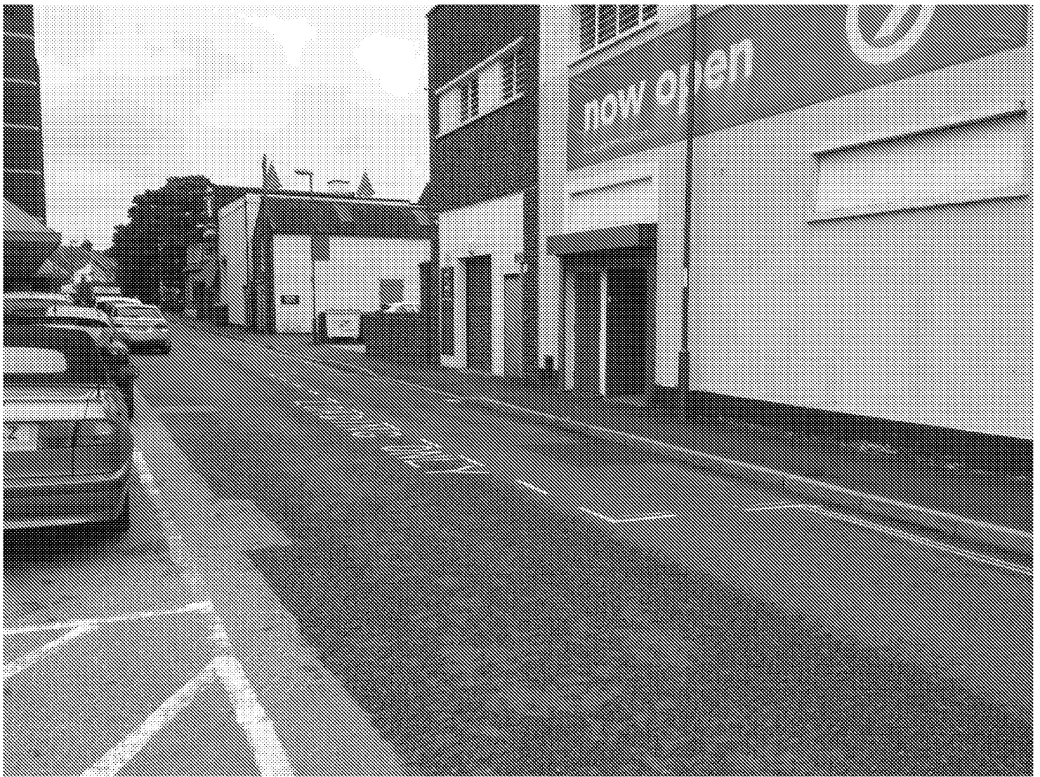
Photo 1: Loading Bay on Bedford Road
