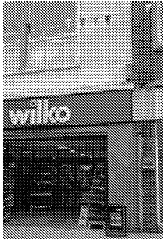
Front Entrance materials.
