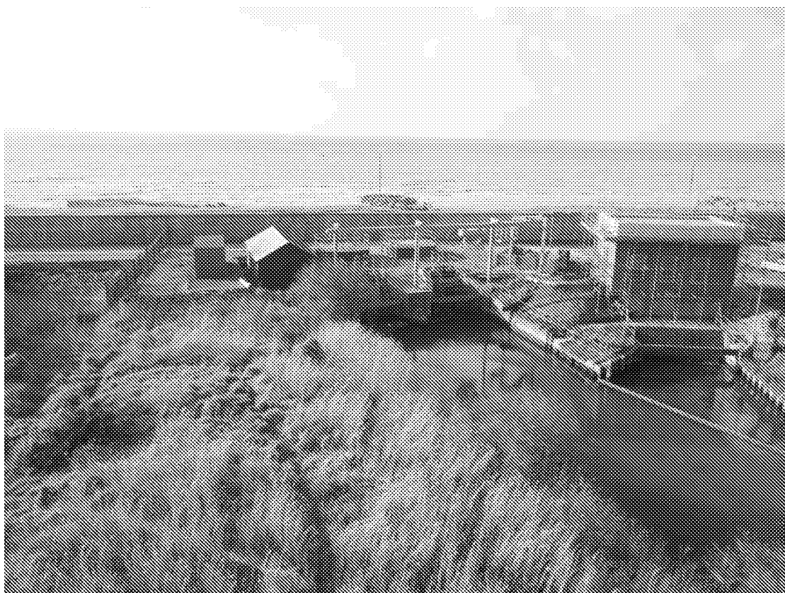
Figure 4: Pumping station and sea wall defence at Elmer
