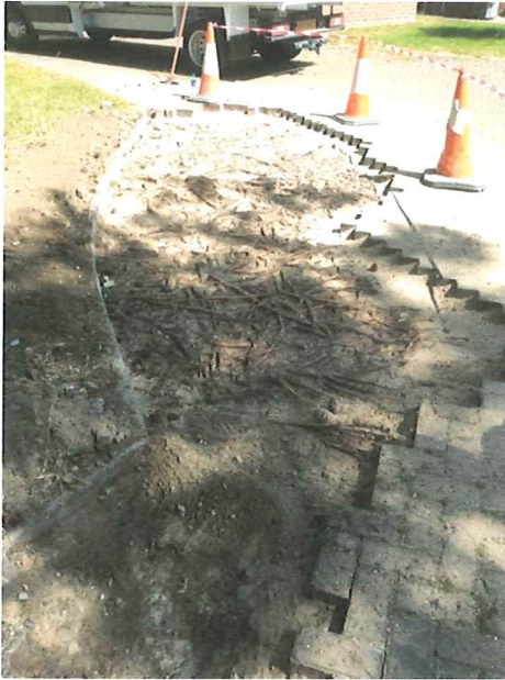
Brick setts lifted and an extensive mass of surface roots exposed. Size 10mm – 100mm
