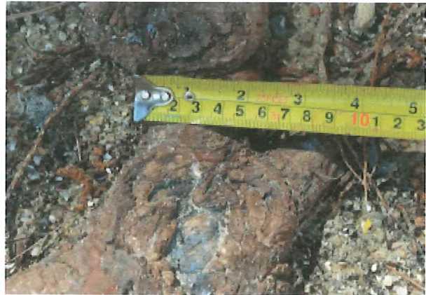
Brick setts lifted and an extensive mass of surface roots exposed. Size 10mm – 100mm
