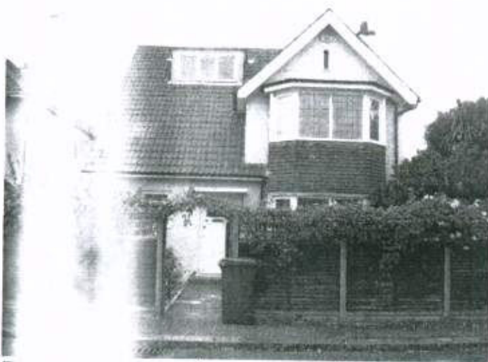
Exterior view on site.
