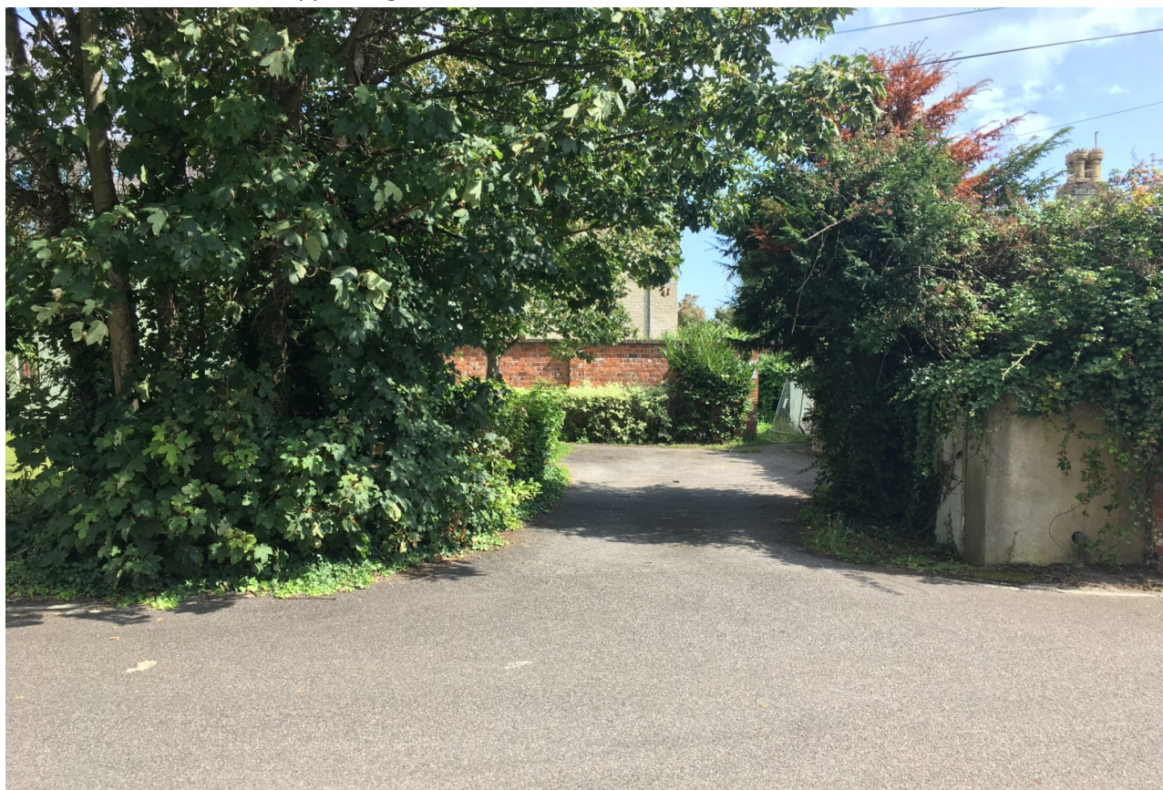
View from access road towards existing boundary wall of courtyard
