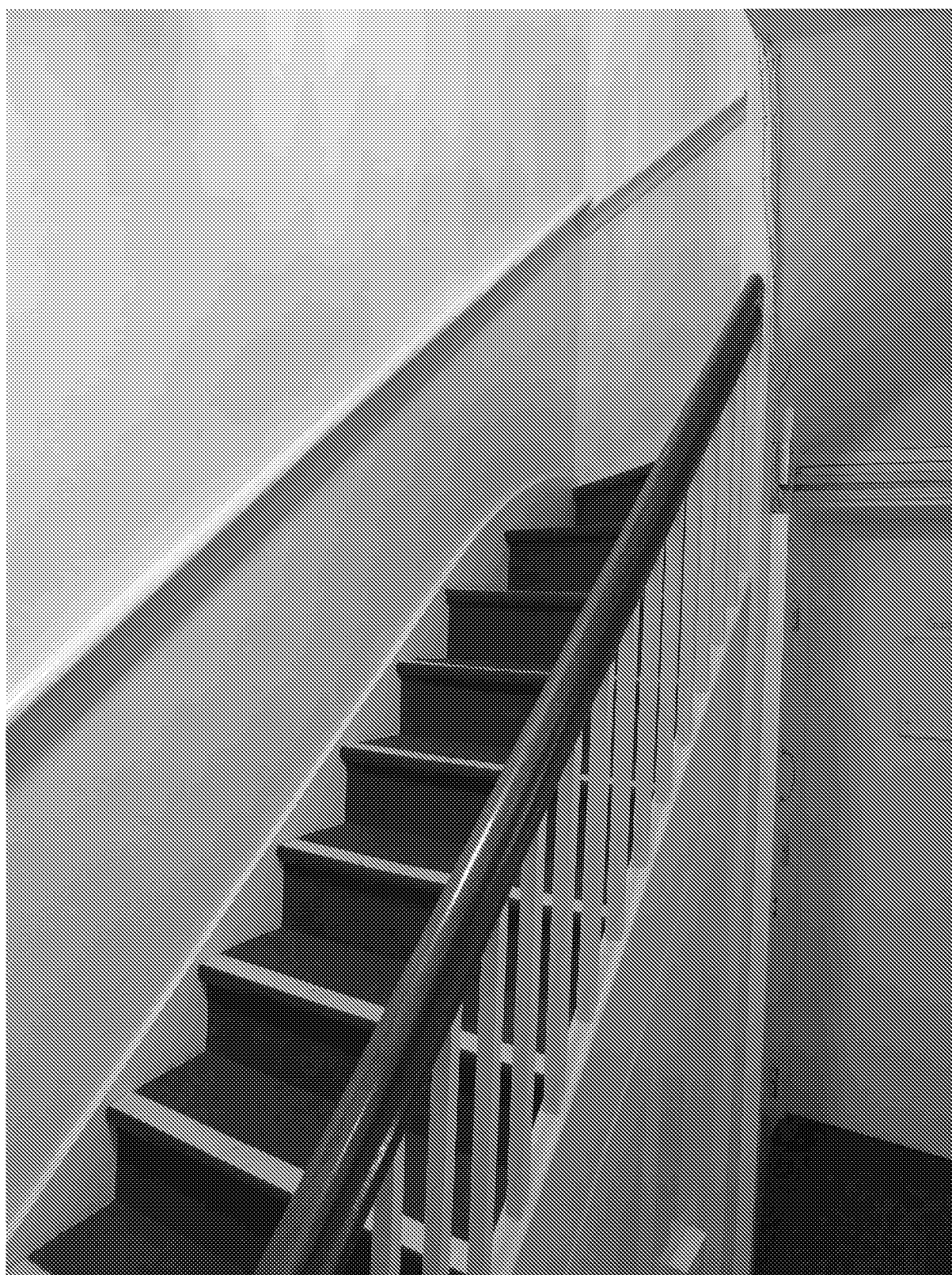
Figure 12: Part of lower flight of staircase up to winder to Charlotte House, 65 Upper Bognor Road
