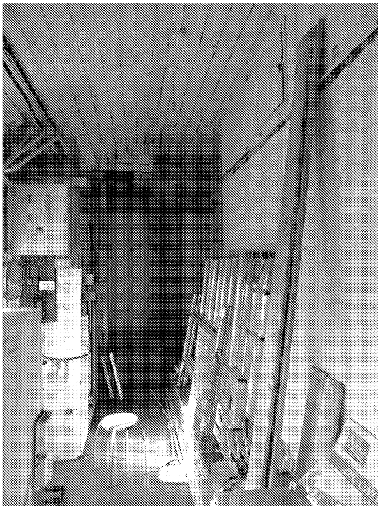
Figure 37: Interior of workshop (unconverted section) to east side of No.71 Upper Bognor Rd
