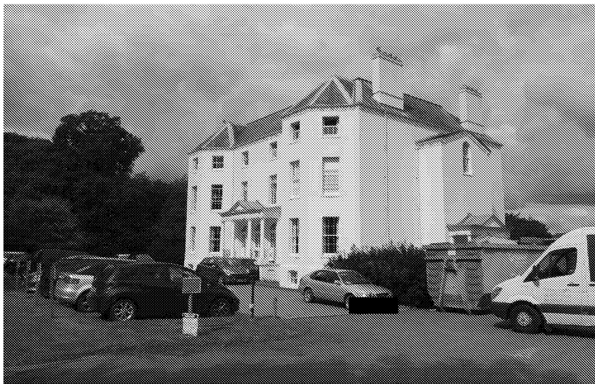
Figure 1: No.53 Mordington, Upper Bognor Road – south elevation
