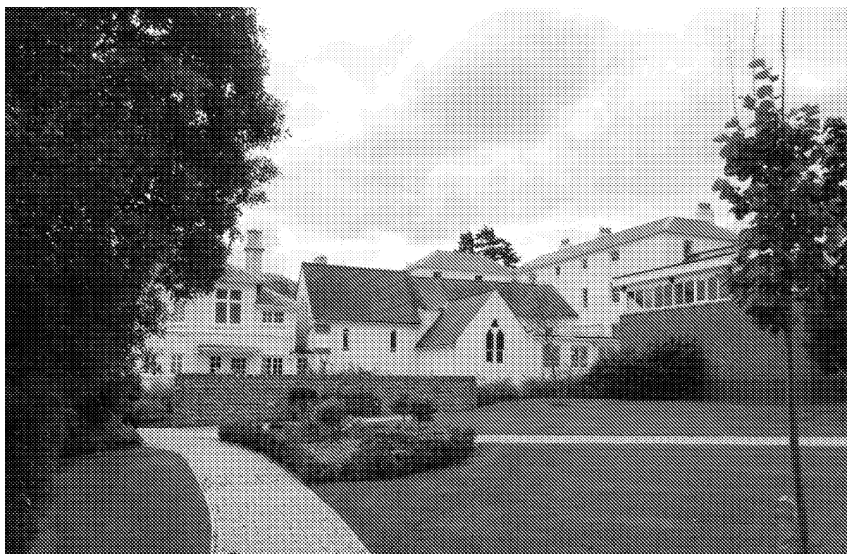
Figure 4: No.57 St Michael's House, Upper Bognor Road – chapel and north elevation
