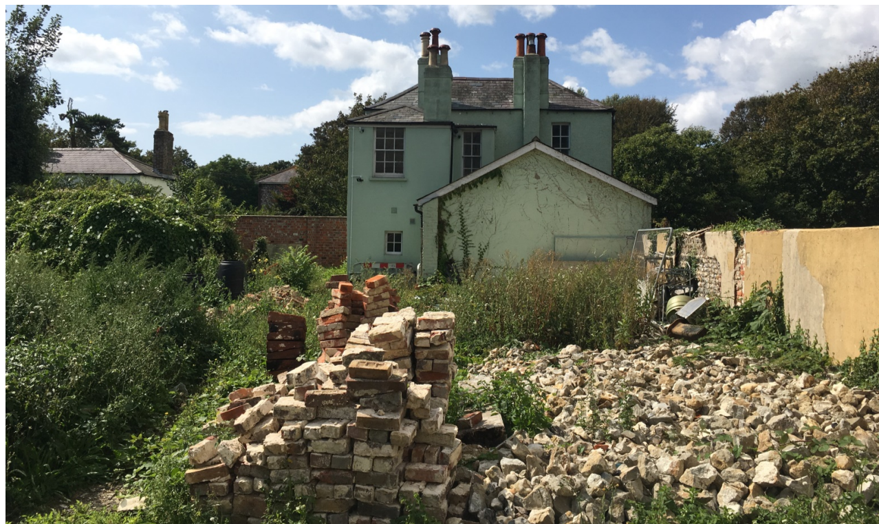
East elevation and setting
