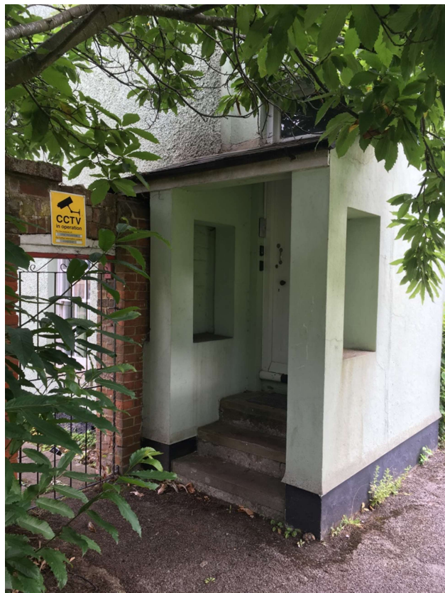
North Entrance to 71A UBR (first floor)
