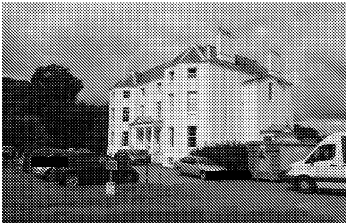
Figure 1: No.53 Mordington, Upper Bognor Road – south elevation
