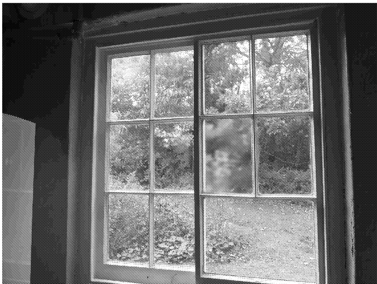
Figure 16: 'Yorkshire' sliding sash to rear outshut/extension to Charlotte House, 65 Upper Bognor Road
