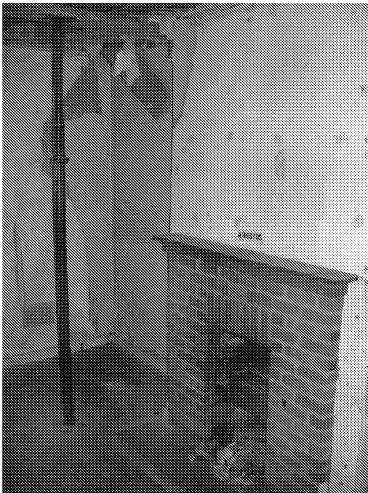
Figure 23: Fireplace, to ground floor living room of No.67 Upper Bognor Road
