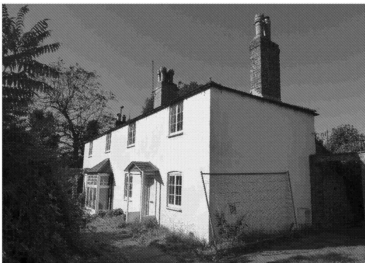
Figure 18: Nos.67 and 69 Upper Bognor Road – east and north elevations
