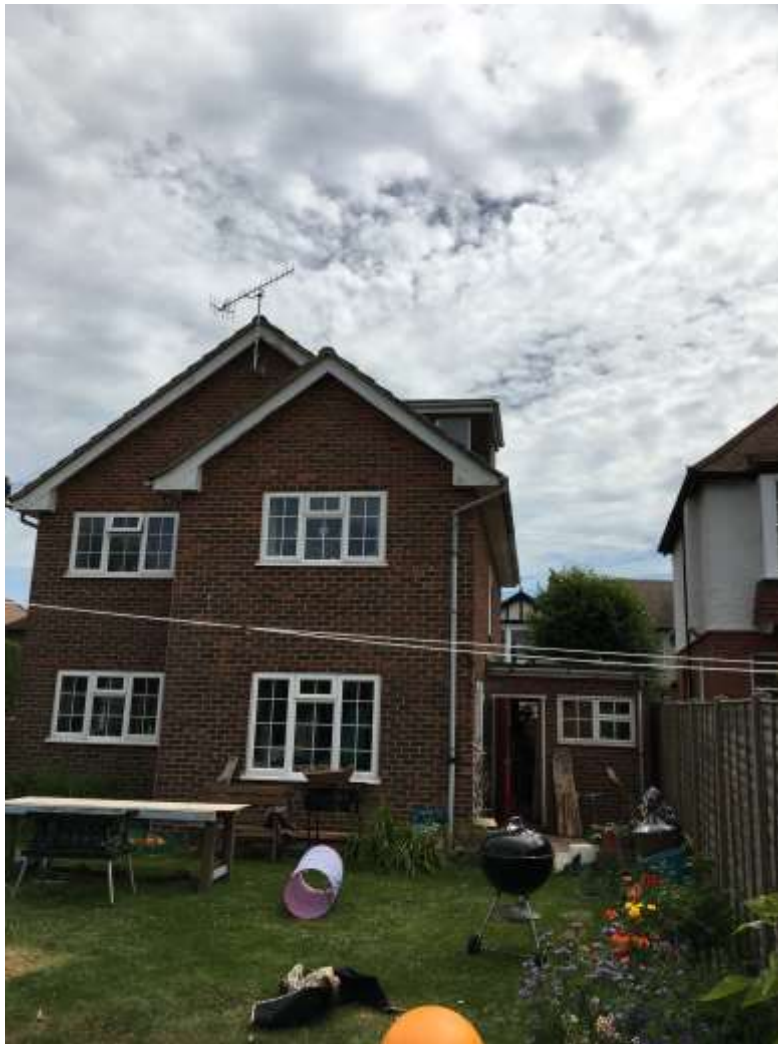
Photograph 01 - Showing the existing rear elevation.
