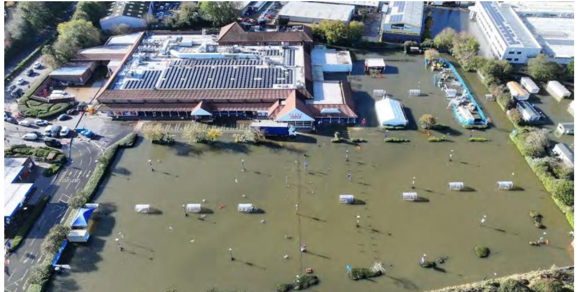
Flooding at Tesco during the 2023 flood event ((image obtained from the West Sussex County Council S19 Flood Investigation report)
