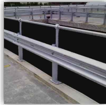
3. 1100mm high handrails incorporating armco barriers and opaque infill panels
