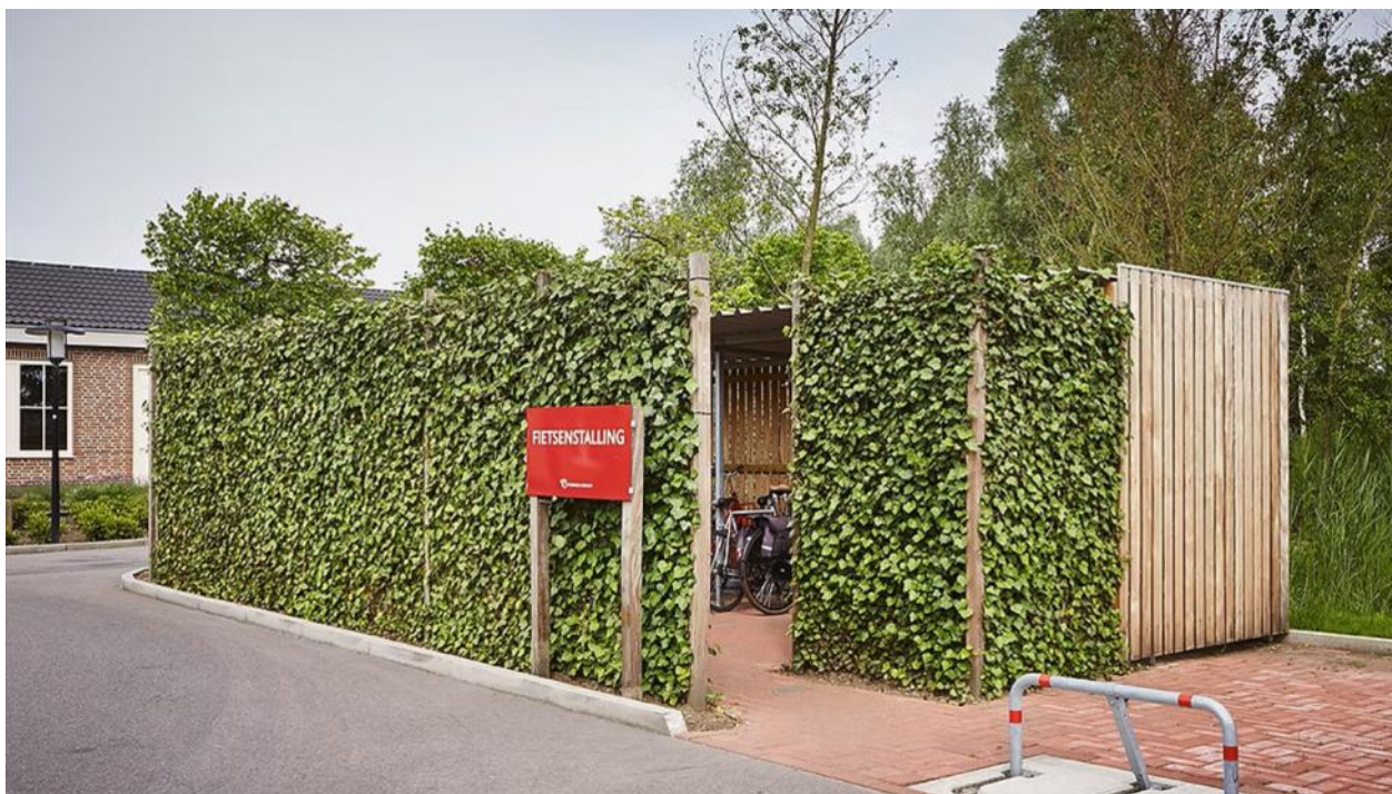
7. Landscape shielding and timber access gates
