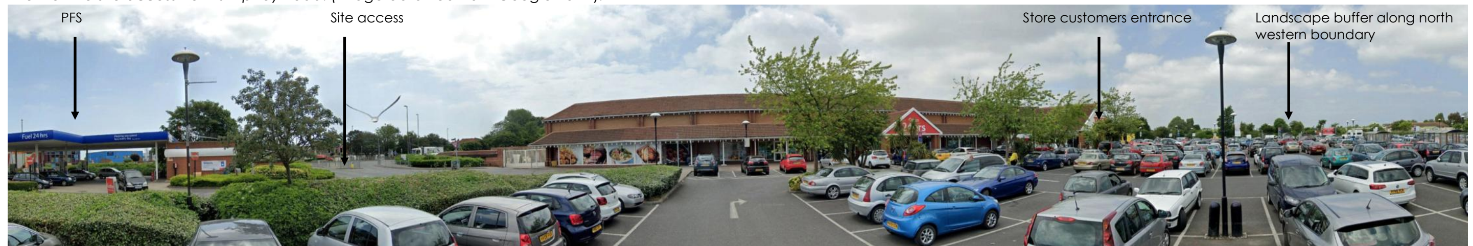
View of the main store frontage and its relation with the site access, PFS and car park. (Image obtained from Google Earth).
