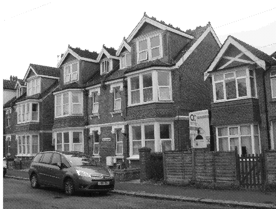
Above: Front view of the application site building, facing north, onto Richmond Avenue, depicting the property's material character, architectural quality, mass, scale and composition relative to adjoining properties. See also cl. 2.2.3
