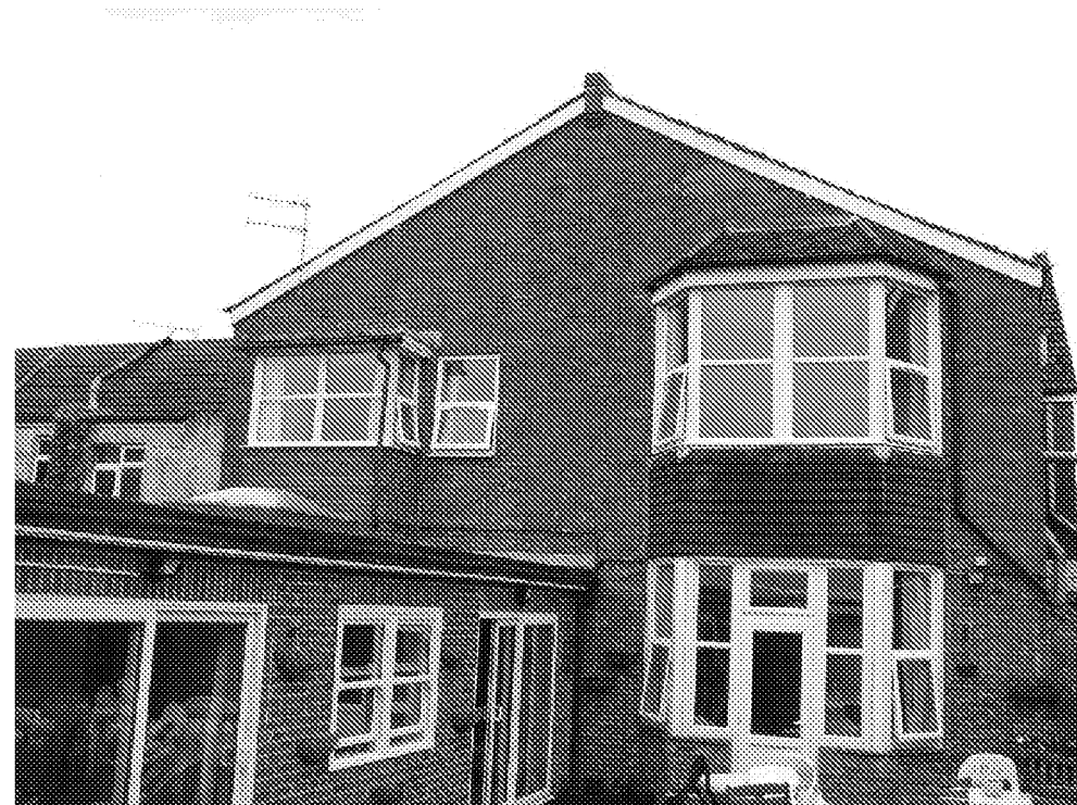
Above: The rear of the Rest-home building facing south into the rear amenity courtyard garden depicting the informal arrangement of windows, architectural character, and the rear single-story extension.
