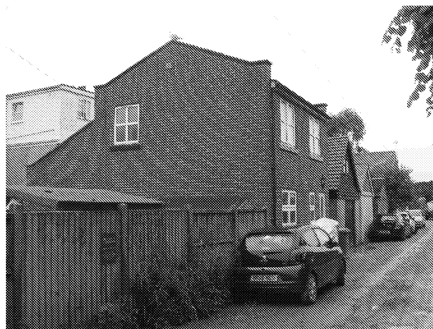
Above: View of the rear vehicular pathway with a typical 2 storey outbuildings facing the pathway. See also cl. 2.2.2
