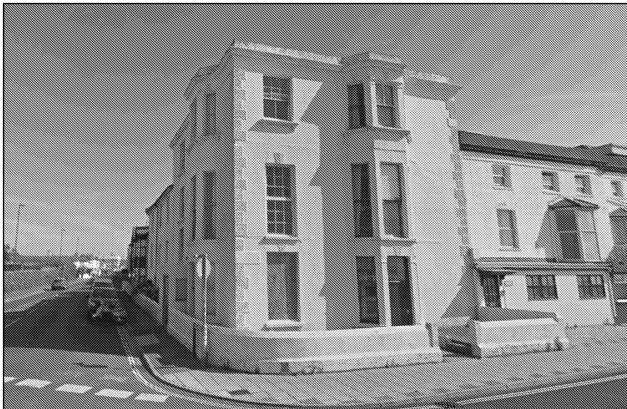
Front (southern) elevation.
