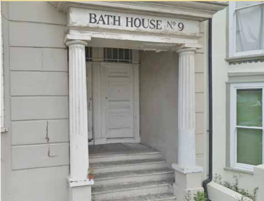
9 The Steyne, PO21 1TX
