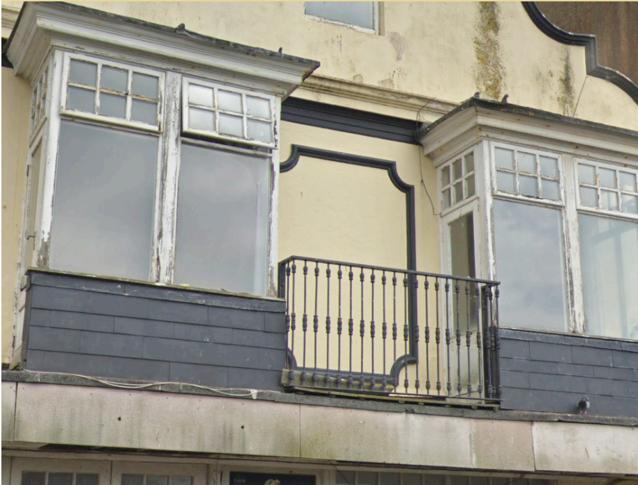
4 Waterloo Square, PO21 1SU
