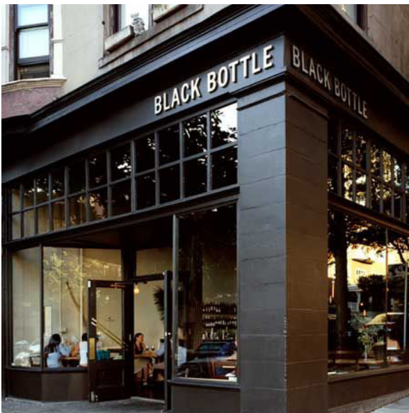
Retail at ground floor level with larger windows opening onto street
