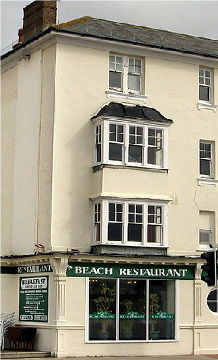
The Former Beach Hotel before demolition
