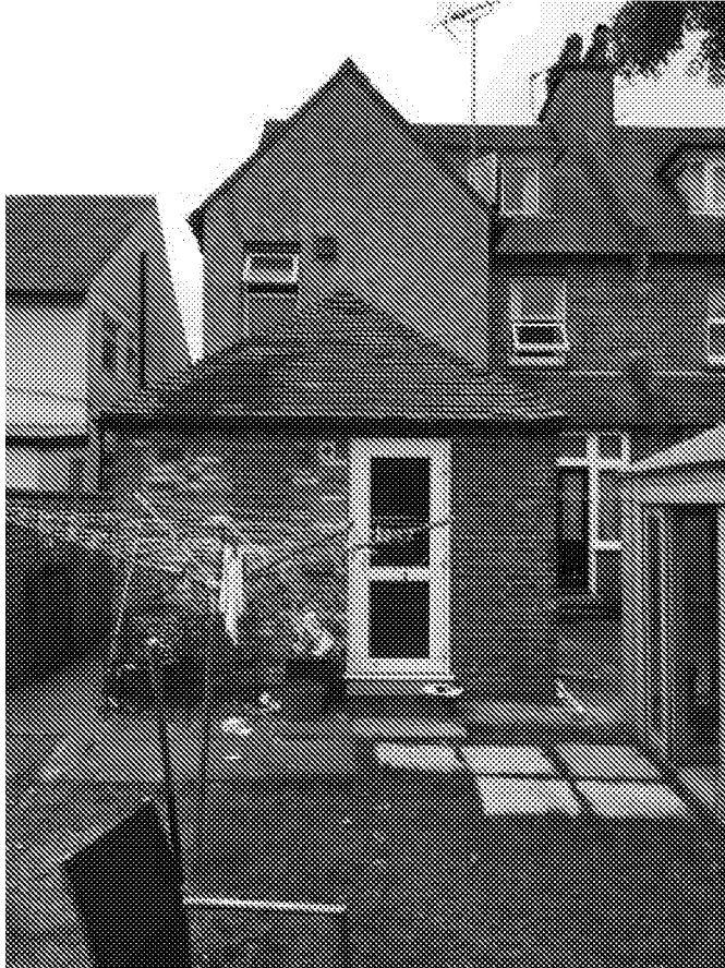
Photograph 01 - Showing the existing North West Elevation.
