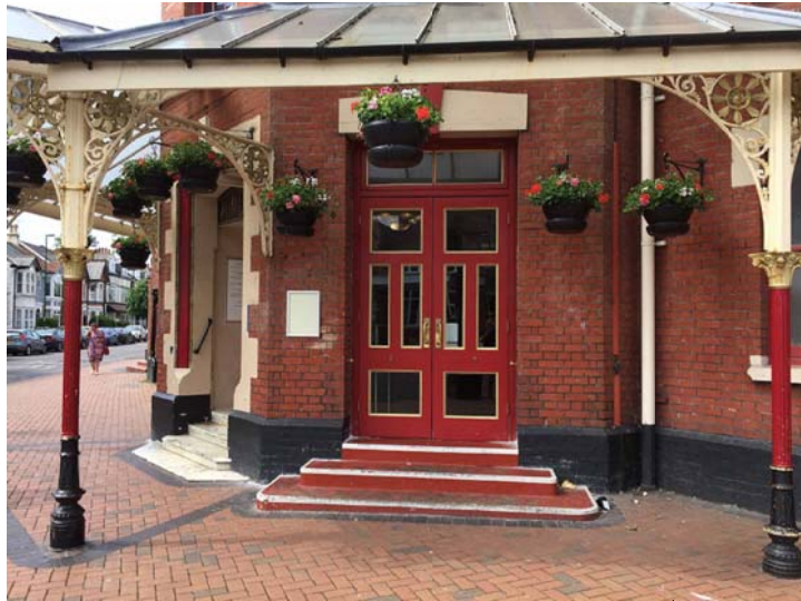
EXISTING FRONT DOORS AND STEPS
