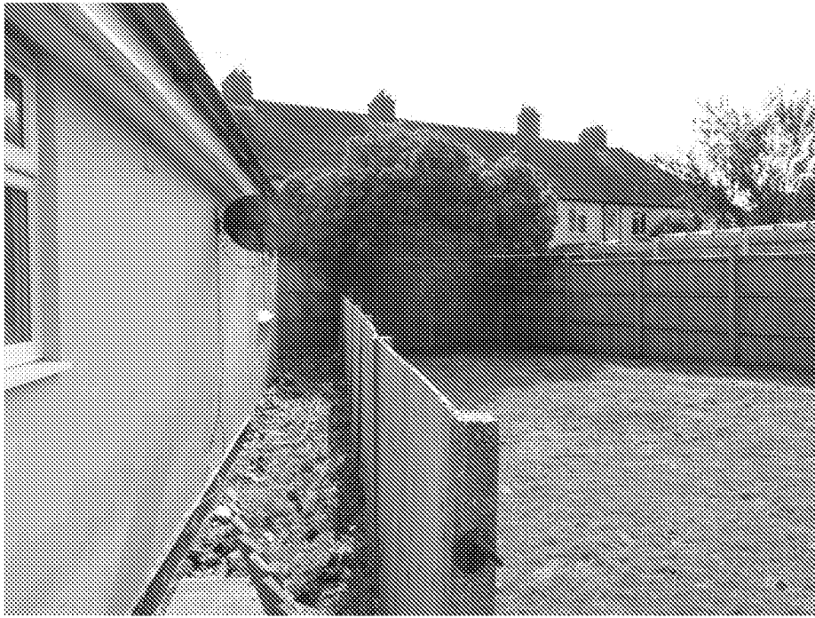
7 – Rear of Cottage 2 with boundary fence
