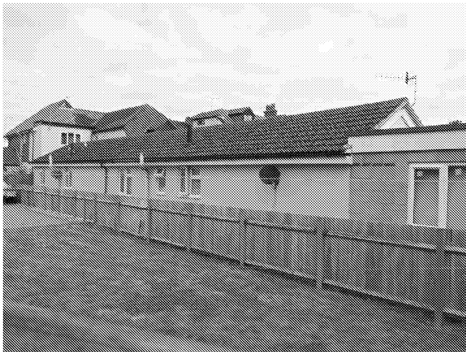
6 – Rear of Cottage 2 where new patio door to be located
