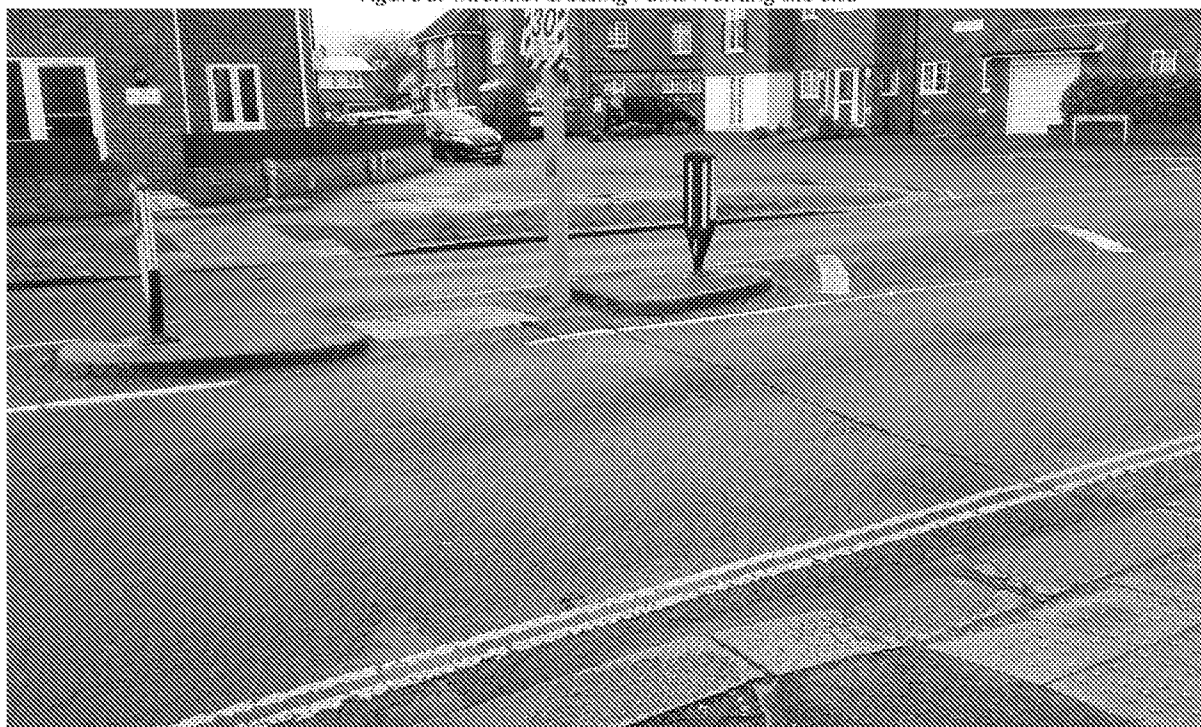
Figure 5. Informal Crossing Point Fronting the Site
