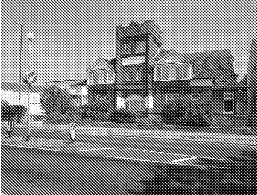
Fig 5: Existing building from Aldwick Road
