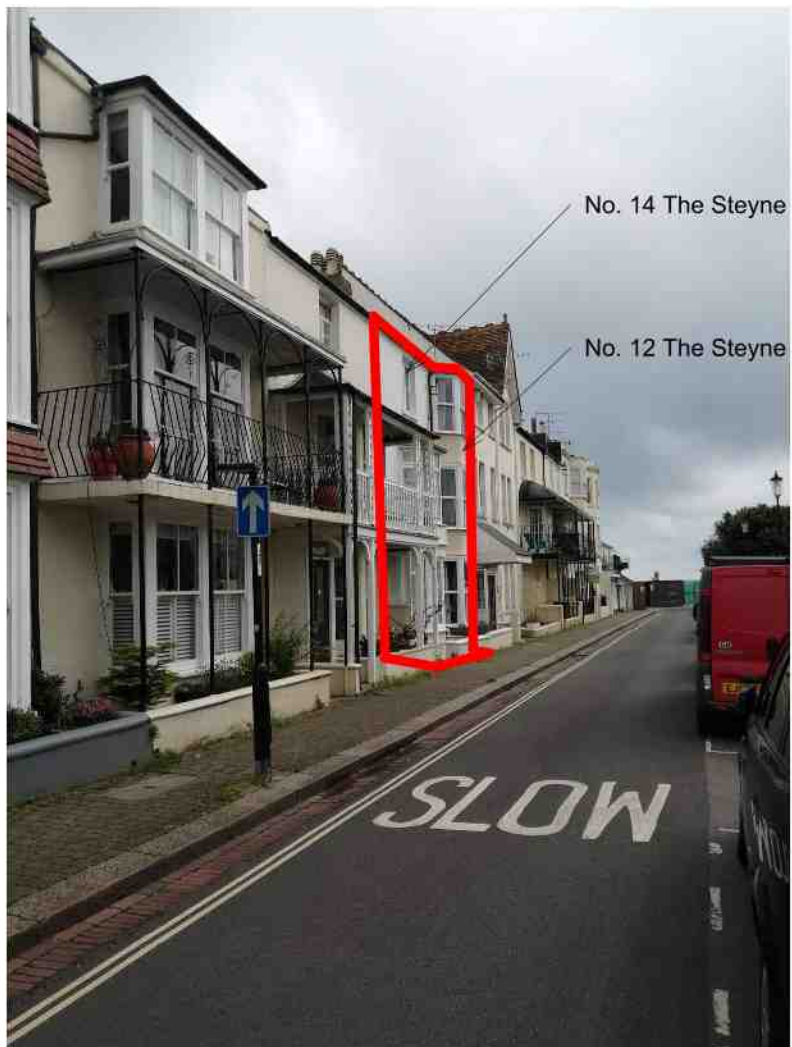
Examples of Neighbouring Balconies Similar to Proposed at 14 and 12 The Steyne
